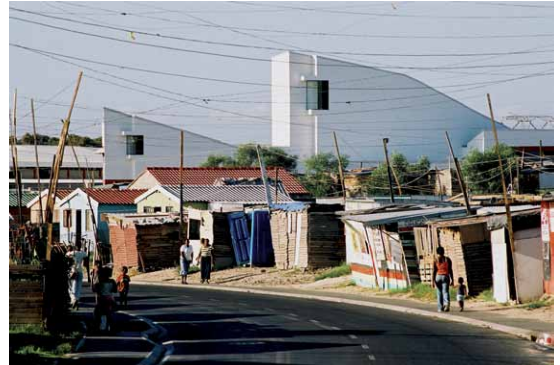
Inkwenkwezi Secondary School (2007), Cape Town , by Noero Wolff Architects (photo Heinrich Wolff)
